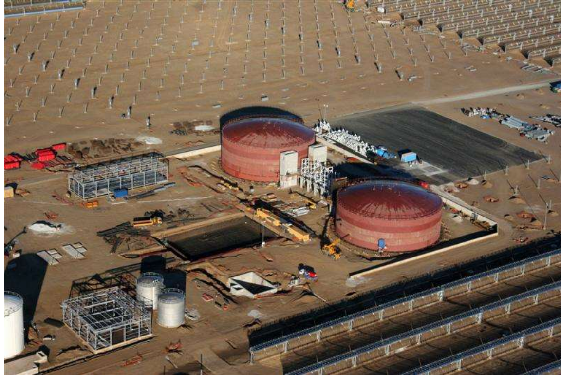
(about 30.000 tons of molten salt for 8 hours of 50MW el production)
